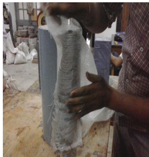
Fig.2-fixing up GFRP sheet on column
