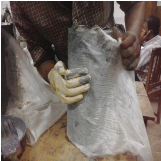
Fig.3-fixing up GFRP sheet on column
